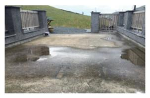
Any small cracks and damaged areas can be repaired with Tecnoband reinforcing mat embedded in a coat of Desmopol membrane (AFTER PRIMING). Any significant cracks to be filled using Desmoseal PU Mastic or any approved Polyurethane based mastic, (BEFORE PRIMER IS APPLIED). AVOID the use of silicone based mastics.
