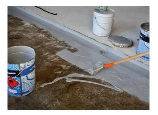
When first opening Desmopol tins, the product must be stirred thoroughly ensuring any settlement at the bottom is mixed in. Desmoplus Accelerator is then added at the exact ratio of 110ml (of Desmoplus Accelerator) per litre of Desmopol (or 2ltr/25kg tin or 500ml/6kg tin of Desmopol) and mixed at a slow speed to avoid air entrapment/bubbles. Make sure the Desmoplus Accelerator and Desmopol are thoroughly mixed together before applying (should take a couple of minutes).
