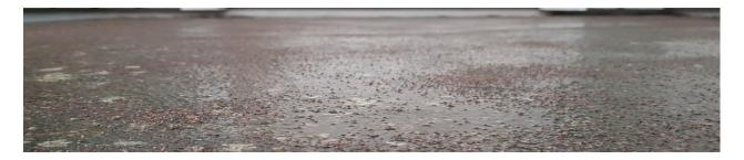
Temafloor PU 0229 grey (Applied @ 0,51/m2 to give about 2mm DFT) + anti-slip white sand @ 0,6-1,2 mm broadcasted on to wet film to fill the surface thoroughly until the surface was covered with loose, unbonded aggregate at a spread rate of approximately 6kg/m2
