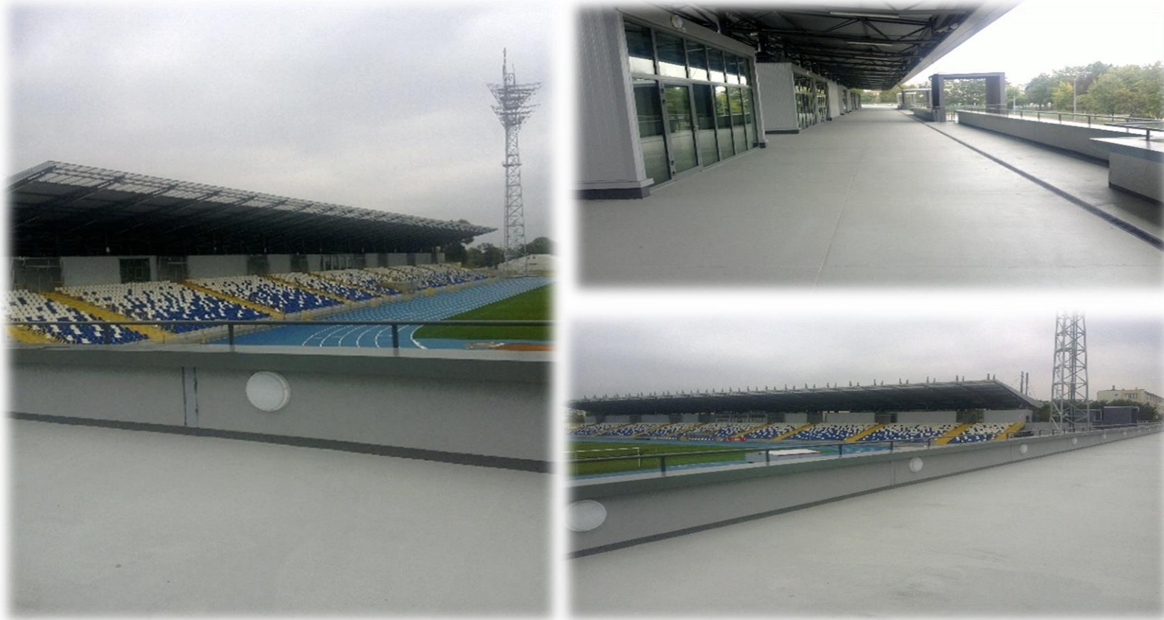
Stadium in Mielec, area 4000 m 2 Contractor: PROTECH/KORKOLOR
