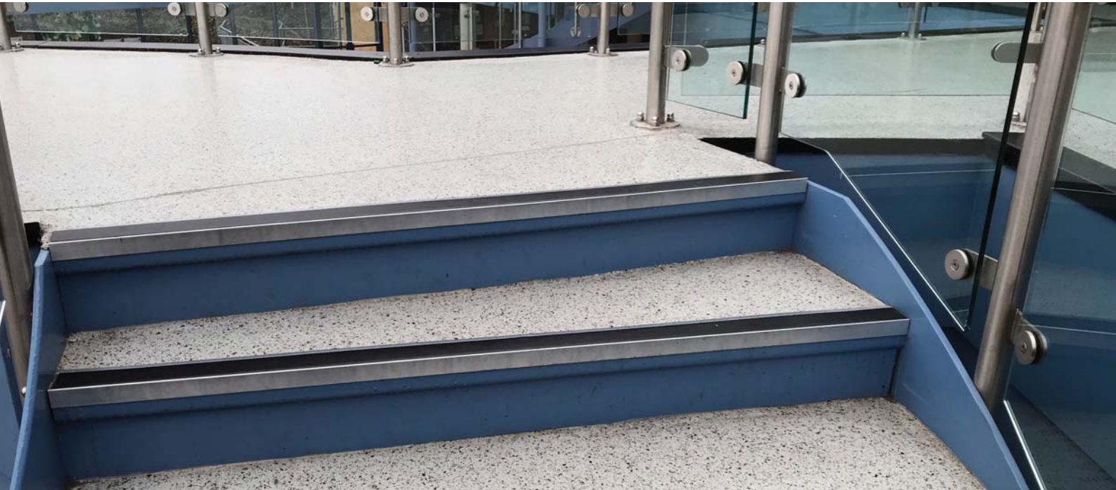
Resucoat Deco Flake SF – finished working system. Education facility, United Kingdom.
