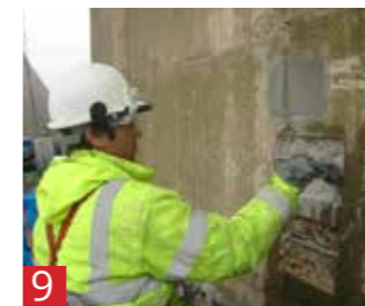
9 Cathodic Control Restricting the access of Oxygen to the cathodic site by coating the steel.
