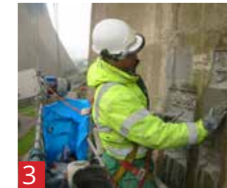
3 Concrete Restoration Repairing or replacing concrete using a variety of mortars.
